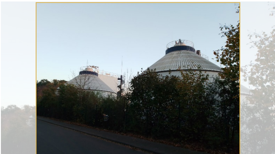
Figure 25. Sewage Treatment Plant.
